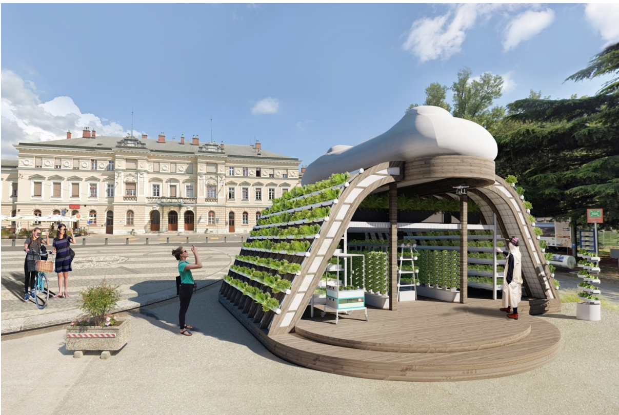
MFC toilet structure made from recycled wood, incorporated into a precision gardening unit with robot-farmed hydroponically grown plants. Concept for Nova Gorica GO! 2025 festival, rendering by Anna Vershinina, 2023.
