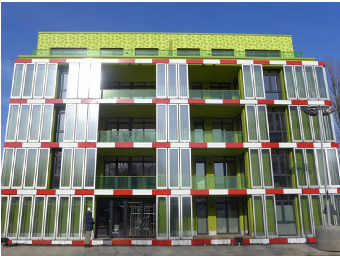
BIQ House, the world’s first building powered by algae, Hamburg, Germany, courtesy of Colt International, Arup, SSC GmbH, 2011.
